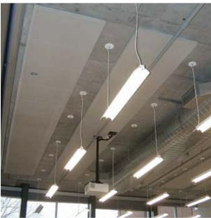
PHONSTOP™ direct-apply, glue-up wall and ceiling acoustic panels are produced from 100-percent recycled glass granules fused together to form rigid, lightweight, fiber-free sound absorbers suitable for interior and exterior applications. PHONSTOP absorbs sound energy within its open-cell, sintered glass core resulting in exceptionally high noise reduction over a broad frequency range, controlling excess sound reflection and reverberation.
